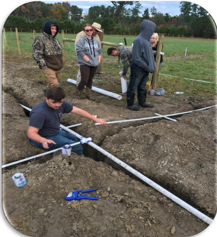
Constructing Waterlines
