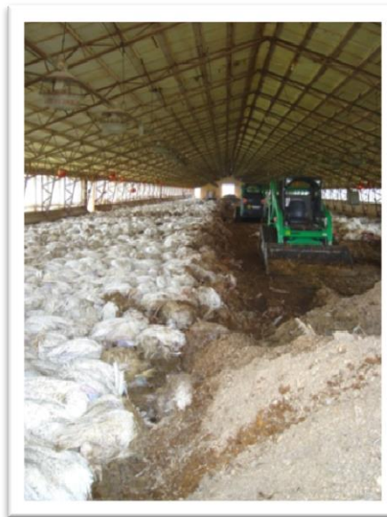
Clearing the base (photo by Gary Flory)
