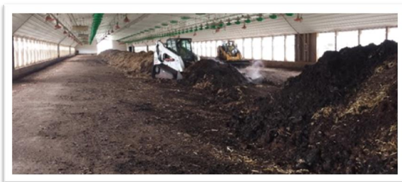
Turning in-house with a skid loader (photo by Josh Payne)
