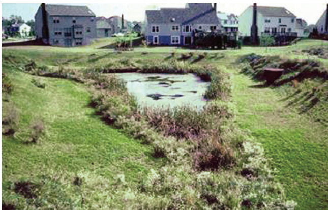
Figure 1. Extended detention pond during wet period (VA-DCR 2011).
