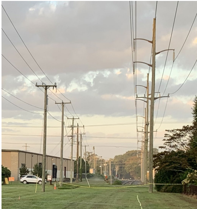
Figure 2. Examples of a distribution power line (left) and a transmission power line (right). Transmission structures typically support more lines and are built taller than distribution structures due to the higher voltage and greater liabilities of a power outage. (Photo by Laurie Fox.)
