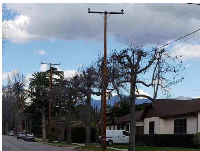
Figure 3. These trees have been topped, which is an inappropriate pruning practice. Water sprouts have grown in response to excessive branch removal and will quickly conflict with overhead utility lines due to their rapid growth rate. (Photo reprinted by permission from Rebecca Latta, rebeccalattaconsulting.com .)
