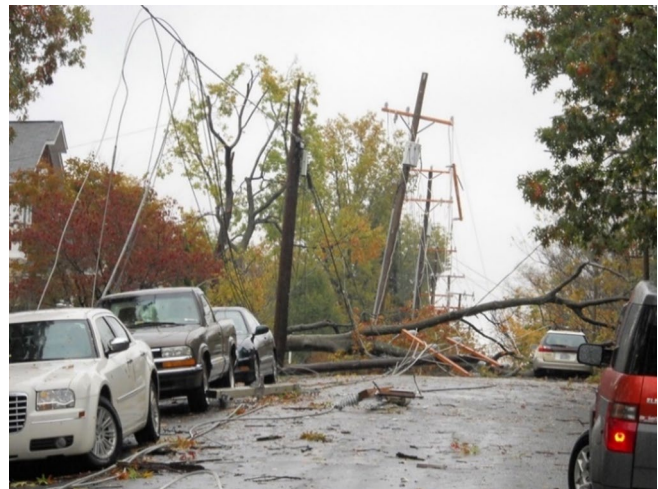
Figure 1. Tree failure damaging utility lines after a storm. (Photo courtesy of Arlington County, Virginia, via Flickr.)
