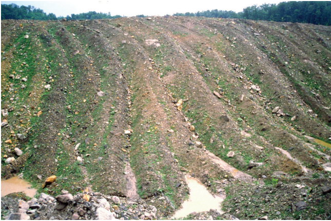
Figure 9. Example of uncompact, roughly graded surface ideal for tree planting.
