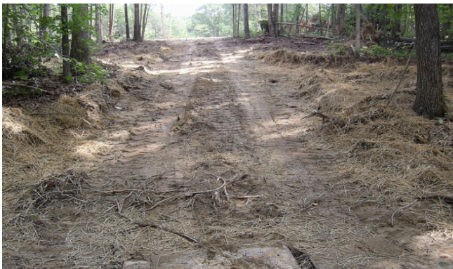
Figure 1. Multiple BMP options are available for closure of temporary stream crossings.
