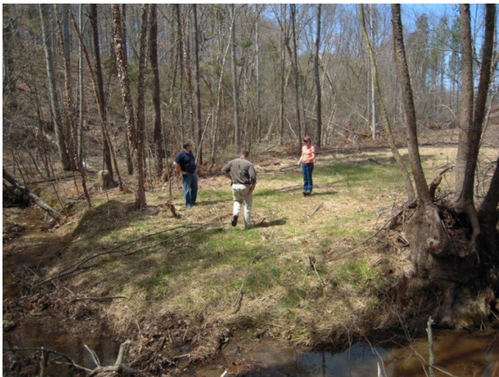
Figure 3. Temporary crossing closure with “mulch” (water bars, seed, lime, fertilizer, straw mulch).
