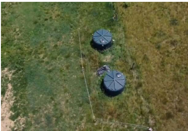
Figure 5. Overhead View of Two Plastic Reservoir Tanks
