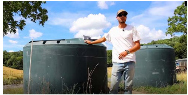
Figure 6. Host Farmer Demonstrating Reservoir Storage at System High Spot to Enable Gravity Flow to Stock Tanks
