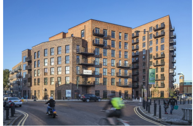
Figure 7: Dalston Lane, the Largest CLT Building in the World. Source: (Schuler Timothy A., 2018)
