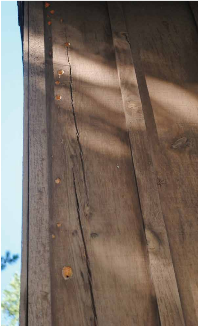
Figure 5: Illustration of damage typical of that inflicted by foraging woodpecker. (Photo is licensed under CC BY-NC-ND 2.0 dianecordell)
