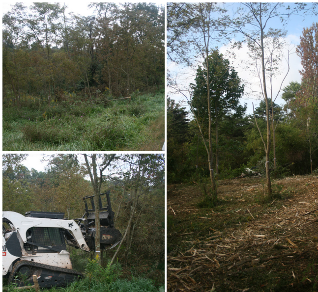
Figure 5. Mulching is a good way to clean up a site quickly and with minimum disturbance (as compared with bulldozing), but the benefits must be weighed against generally greater expense. (Photos by John Fike.)
