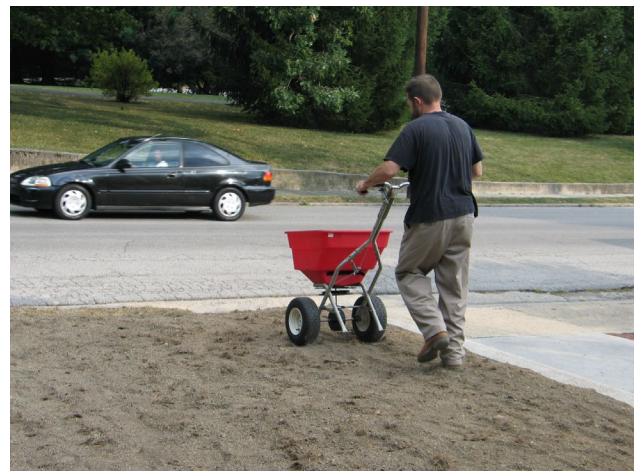
Figure 1. A complete renovation is in progress on this lawn with the removal of all previous vegetation, soil tillage, and seeding of an improved cultivar.
