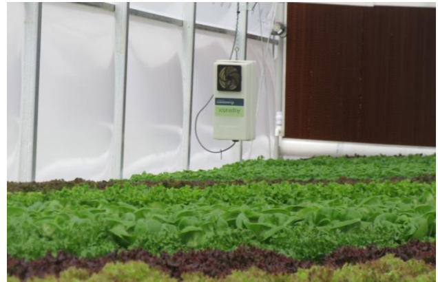
Figure 1. Using an aspirated thermostat, hung near canopy level, helps to accurately control greenhouse temperature. (Joyce Latimer, Virginia Cooperative Extension)
