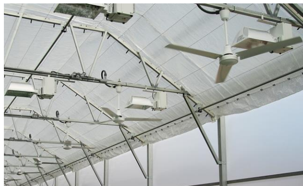
Figure 6. For head lettuce production, paddle fans direct more air into the centers of the heads, improving transpiration to reduce tip burn. (Joyce Latimer, Virginia Cooperative Extension)
