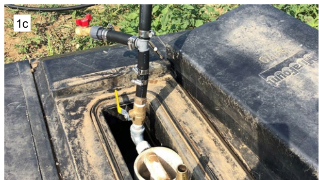
Figure 1. A permanent waterer mounted on runners can be pulled with a four-wheeler (a), a gravity-fed stock tank with a floor-mounted float valve (b), tapping into a pressurized waterer with aboveground PE pipe, extending water service to an adjacent field (c). (Photo credits: John Benner, Virginia Cooperative Extension [1a], Matt Booher [1b], Jacob Gilley, Madison County, Virginia [1c].)
